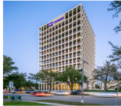
River Oaks Bank Building Houston, TX 170,233 SF Client: L&B Realty
