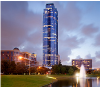
Williams Tower Houston, TX 1,479,764 SF Client: Hines
